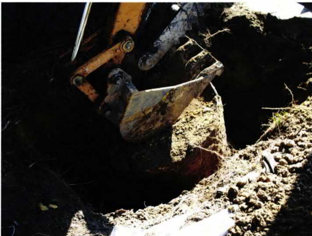
Picture 2: UST 530LaurelBB removal in progress.
